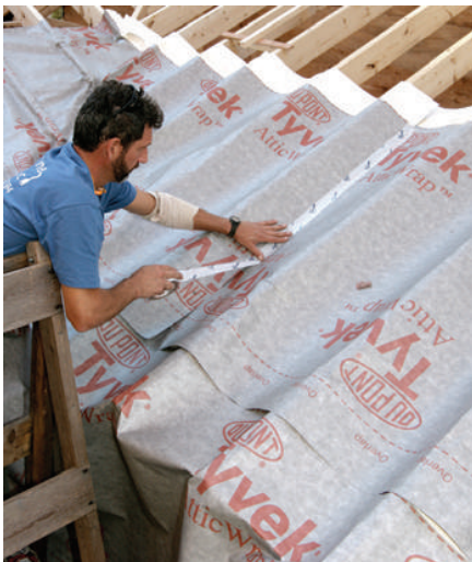
DuPont™ Tyvek® AtticWrap™ is a breathable membrane that helps create a sealed attic system, reducing air leakage and energy loss through the roof.
