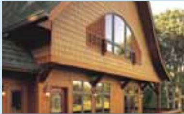
Fiber Cement Siding
